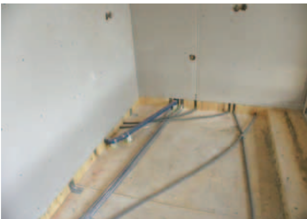
Fig. 68 – Cable routing in floor structure
