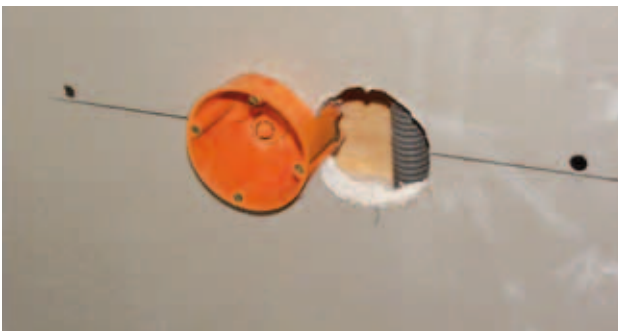
Fig. 52 – Installation of type X gypsum boards by a dry construction worker and socket drilling in the course of that process
