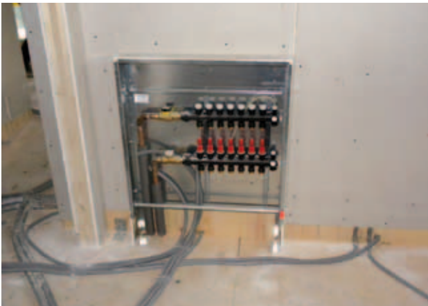
Fig. 66 – Floor distribution cabinet
