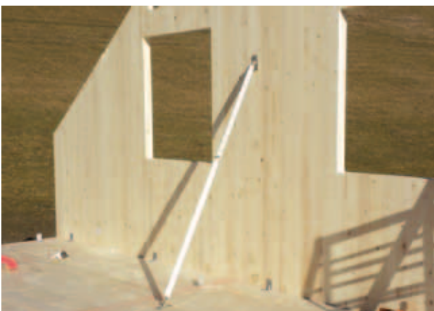
Fig. 1 – Assembly support, positioning bracket
