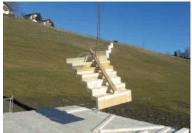
Fig. 48 – Assembly of a prefabricated flight of stairs
