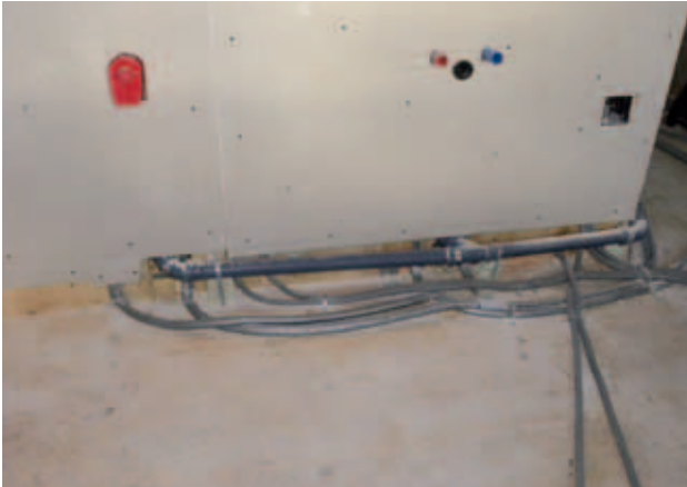
Fig. 64 – Connection of washing machine, washbasin
