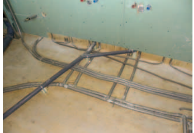
Fig. 65 – Connection of double washbasin
