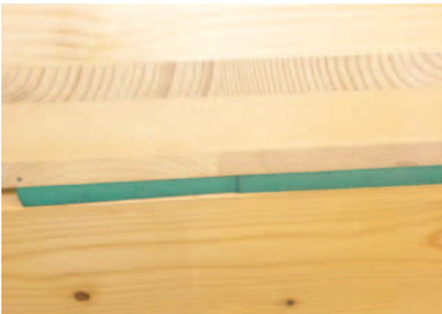
Fig. 14 – Elastomer support, soundproofing layer
