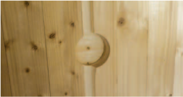
Fig. 50 – Milling grooves for cables
