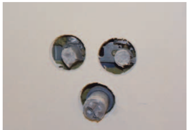
Fig. 69 – Water and sewer pipe connections
