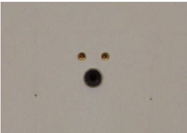
After fastening the installation box, it should be faced with a type X gypsum board and also fastened onto the 5 x 8 cm laths
