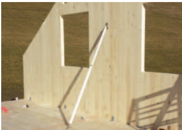
Figs. 43 to 46 – Assembly of KLH® components
