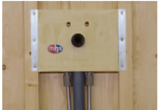
Once the correct height for the water connection and the drain pipe has been determined, the installation box can be fastened on the 5 x 8 cm laths with countersunk bolts
